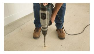
Always use the drill diameter stated in the manufacturer's technical data sheet. Generally, it will be 1/16" or 1/8" larger than the anchor diameter. If the hole is too large, the capacity of the anchor may be reduced. Too small, and it can be difficult to install the anchor and with enough room for the epoxy to form a bond.
