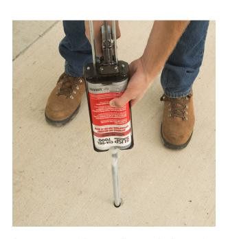
A pure epoxy offers excellent anchoring performance as well as chemical resistance against corrosive chlorine, but its slow cure rate makes it prone to sagging. Pure epoxy would be ideal for the downward installation, shown, of an anchor bolt in dry concrete, yielding best-inclass strength.
