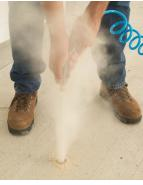
Most manufacturers recommend the hole to be blown out and cleaned with a specific brush. These brushes also serves to roughen the interior surface of the hole for increased bond strength so using the recommended diameter is important. Always drill, blow, brush, blow, brush, and blow.
