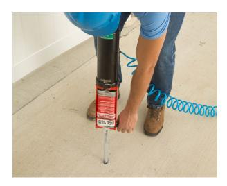
**Not all epoxies are alike:** Types and resulting performance vary widely among epoxy choices and their applications, and product features including nozzle time, gel time, load time, sag, cure time, and chemical resistance will affect how to match the epoxy to the task.
