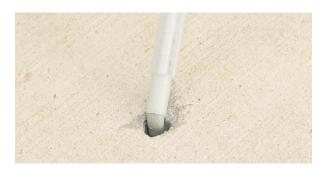
**Nozzle Time**, typically ranging from 3 to 15 minutes, depends on the epoxy type. It is the amount of time that the mixing nozzle can remain inactive with epoxy inside of it and still be able to dispense epoxy for the next anchor. Exceed the working time does not impact the integrity of the epoxy in the cartridges, it just means you need to install a new (empty) mixing nozzle because the epoxy in the nozzle began to cure.
