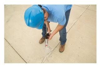
There are specific epoxies for crack repair which can provide either cosmetic non-structural repairs or structural repair via crack injection. Ensure you choose the correct product for your type of repair.
