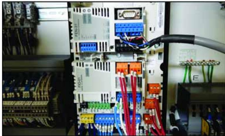
4. Gather the wires toward the bottom of the VFD. This keeps them from interfering with the cover.
