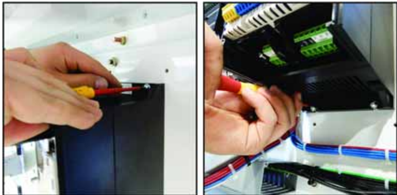
Figure 14: Tightening Mounting Screws
