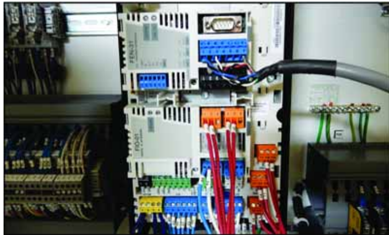
Figure 19: Wired VFD
