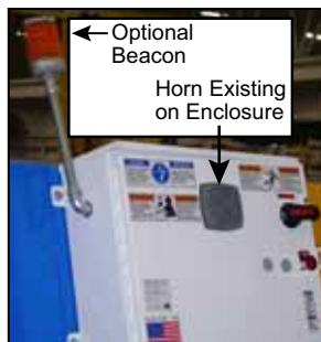
Figure 1: Beacon Added to Existing Finish Roller Enclosure
