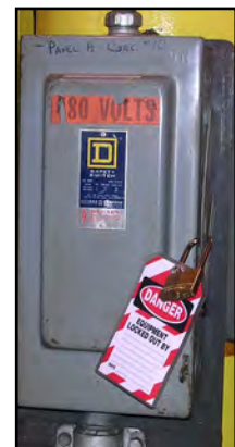
Figure 1: Example of Power Source Locked Out
