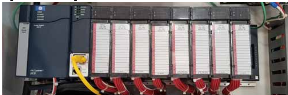
Figure 15: Checking the PLC
