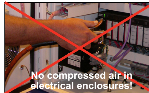
Figure A-1: Never Use Compressor Air Inside an Electrical Enclosure
