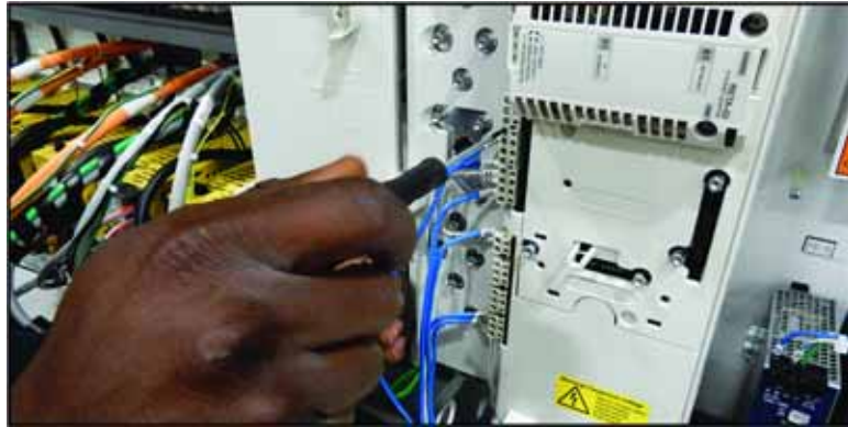
Figure 8: Removing Wires on the Front of the VFD
