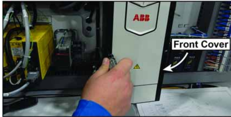
Figure 22: Replacing the Front Cover
