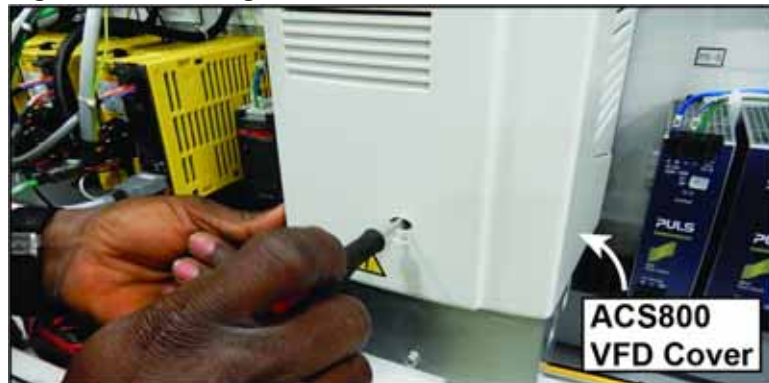
Figure 3: Removing the Cover
