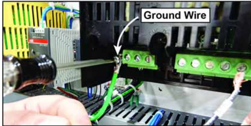
Figure 13: Connecting the Ground Wire
