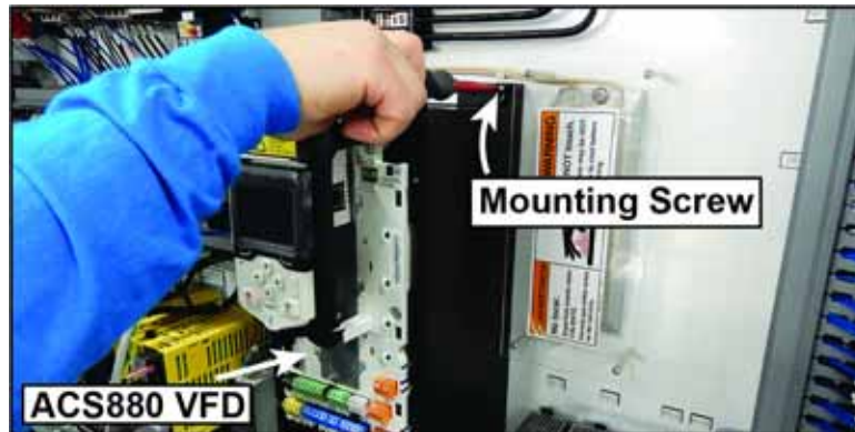
Figure 12: Tightening Mounting Screws
