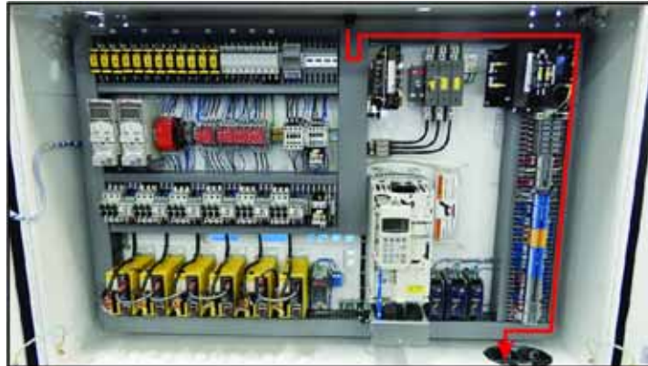
Figure 10: Wire Path (Top Half)
