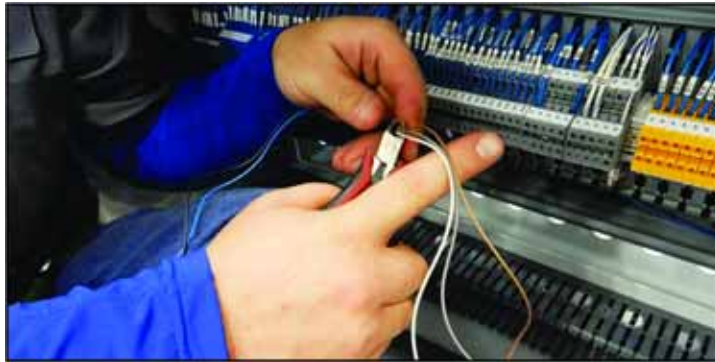
Figure 13: Trimming Brown, White, and Gray Cables
