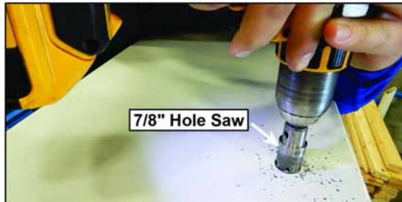
Figure 3: Drilling the Initial Hole
