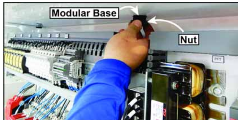
Figure 7: Tightening the Nut
