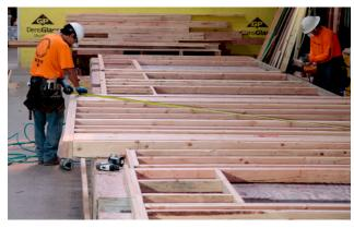
The framing team at Timber Technologies can click on the wall and extract any information about it. Wall height, length, bearing points, header locations, header thicknesses, plate material, you name it. It's all in the
