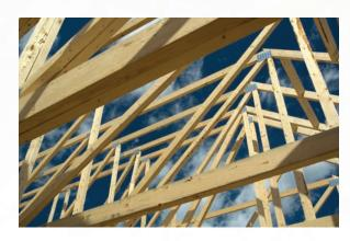
Savvy Homes builds each of its homes in 54 working days, and that cycle time just grew shorter through the use of roof trusses. "Just with what we are saving in roof framing time, we are able to cut our overall framing time by 50%," said Savvy Homes' George Aiken.
